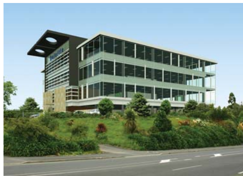
Quadcon's new "green" office building is underway. Deloitte will occupy the Bridge Street development.
