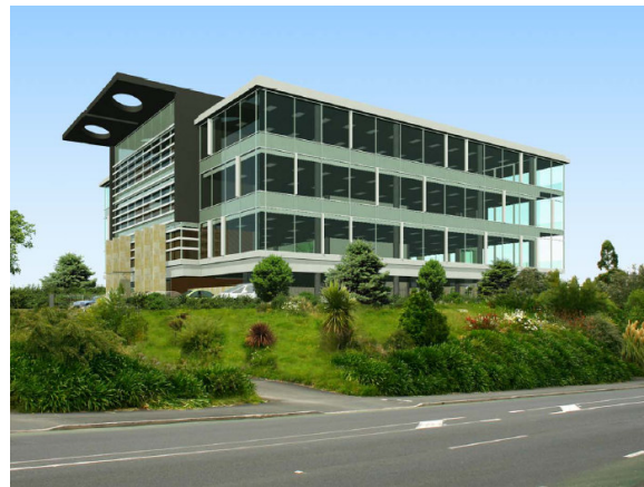
Quadcon's new "green" office building is underway. Deloitte will occupy the Bridge Street development.
